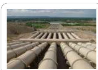
piping planning & inspection
