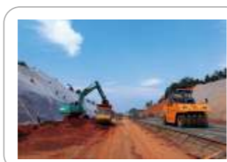
heavy earthwork construction
