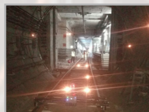
open-cut to shield structure part
