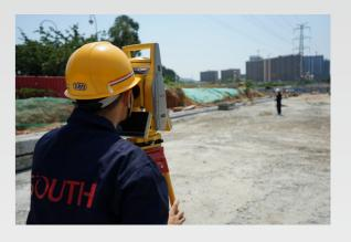
Mission: Plan to stake-out the position of buildings, facilities or roads on the site. Due to the limitation of working environment and the obstacle, most of them are unable to set a RTK rover stably,
