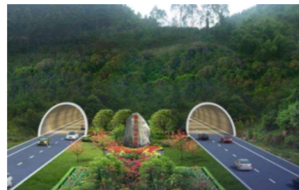
Tunnel Safety Monitoring
