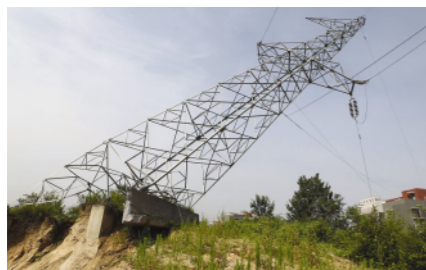
Power Line Tower Tilt Monitoring
