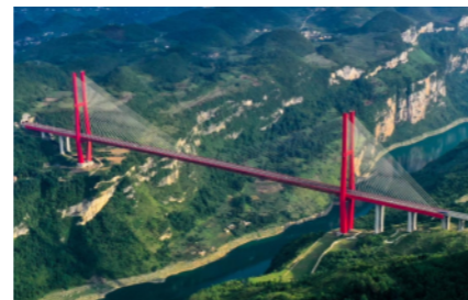
Bridge Safety Monitoring
